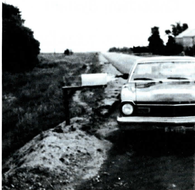
Mailbox stand for "swinging mailbox" comes with two telescoping sections made of regular pipe. Outer pipe has notches welded on it so it can be lifted out with a crowbar if box has to be moved. No cement is needed to secure the vertical post.
