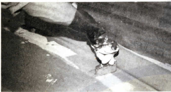
Brushed-on material dries into a rubbery, flexible protective coating that doesn't get brittle with age, unlike tar.
