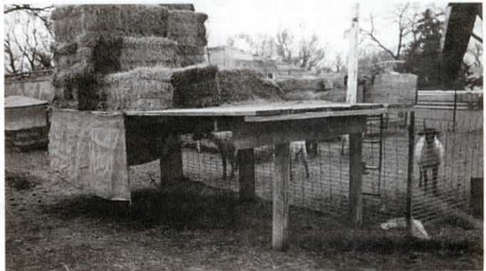
The platform, built out of railroad ties and planks, holds 80 stacked bales.
