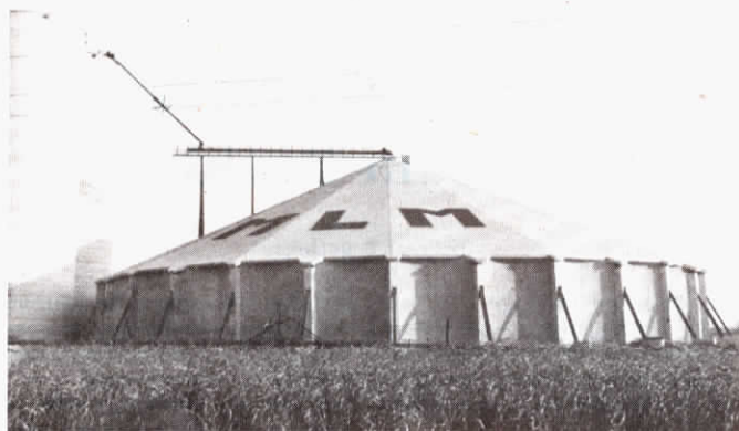
New structure holds up to 1,000,000 bu. and was built at a cost of just 60 cents a bu.
