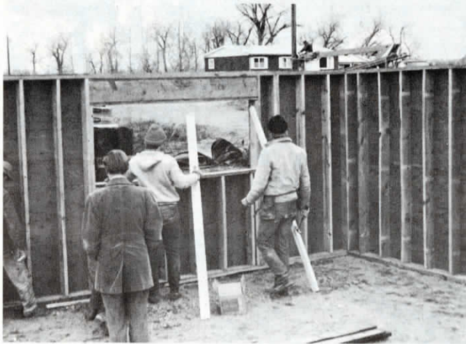
Starting with bare ground, it's not uncommon to have the hole dug and the treated wooden walls up in one day.
