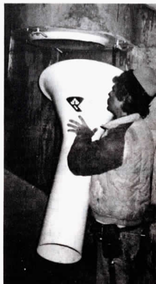
Glendinning's silage-handling funnel fits any silo discharge chute.
