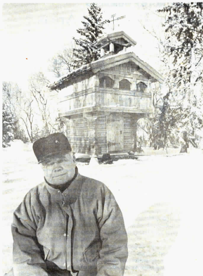
The "Stabbur", constructed entirely with hand tools, is 8 ft. sq. on the bottom level, 12 ft. sq. on the top level, and 22 ft. tall (to the top of the weather vane above bell tower).
