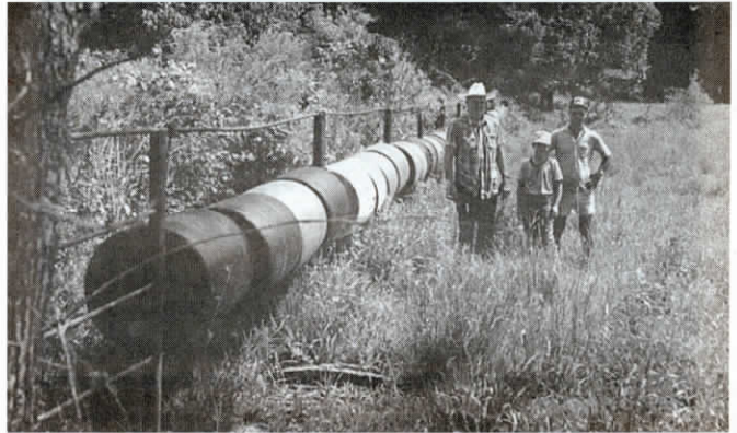
Flood-proof fence made out of 55-gal. detergent drums keeps fence intact.
