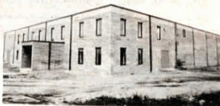
Staves were stacked lengthwise to form 10-in. thick walls.
