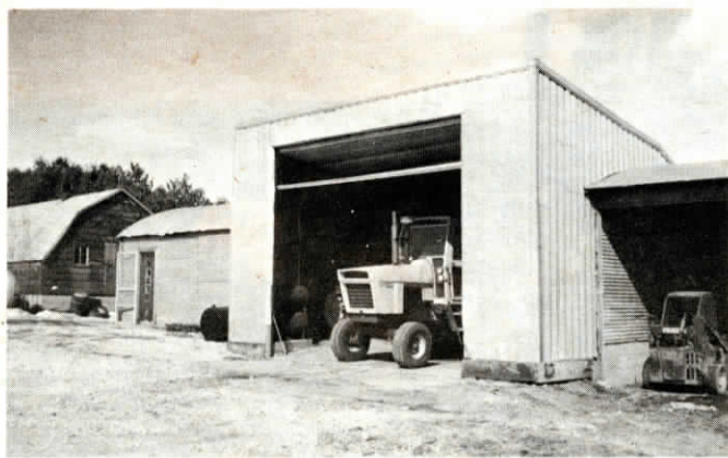
Mensen built a high-ceilinged 18 by 20-ft. shop at the center of the quonset and fitted it with bi-fold doors.
