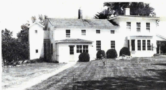
Two story, 6 hole outhouse built along left side of the house has plaster walls and a stone foundation.
