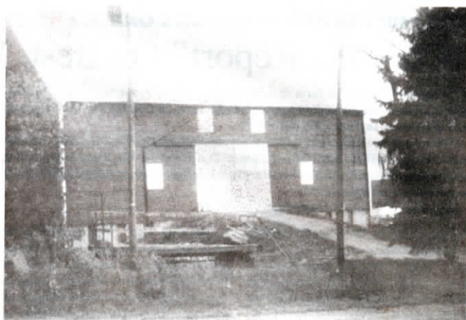
Restored barn is painted red and white. All doors and windows work like new.
