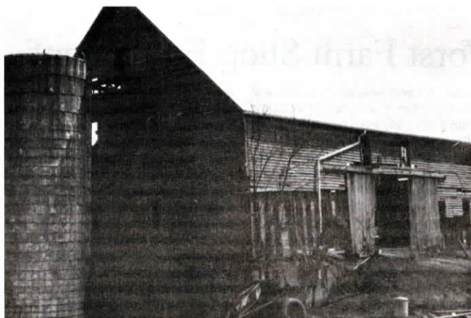
Steepleton totally rebuilt this worn-out barn to its original condition. "We use quality materials and don't cut any corners. We offer true craftsmanship," he says.
