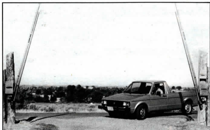
Single solid-state controller operates both 14-ft. sections making up 28-ft. wide gates.
