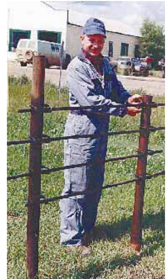
Shamansky shows a steel fence that he built as a sample for customers. He sells a complete package including tubing, sucker rod, and clamps.
