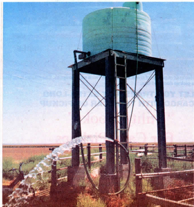
This 1,600-gal. overhead tank is refilled by garden hose. It lets Cook fill sprayer fast without the need for an expensive transfer pump.
