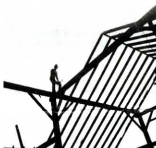
Andre has developed special "short cuts" for dismantling old barns without heavy equipment.
