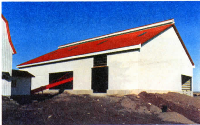
A stacker delivers manure from barn gutters directly into prefabricated building.
