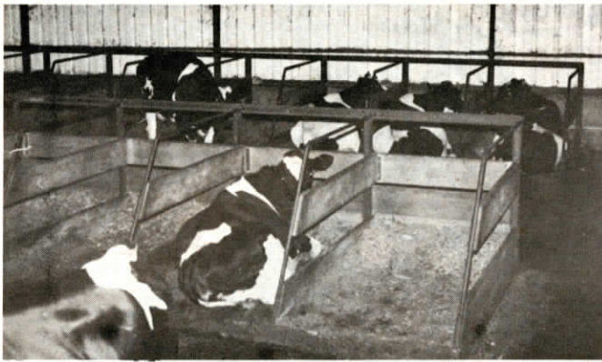
Curbing, partitions and inside wall are all built into the independent stalls which you simply set inside empty barn shell.
