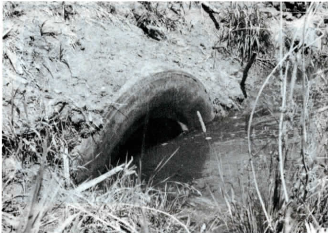
Tires are placed upright, side by side, to form low-cost culvert.
